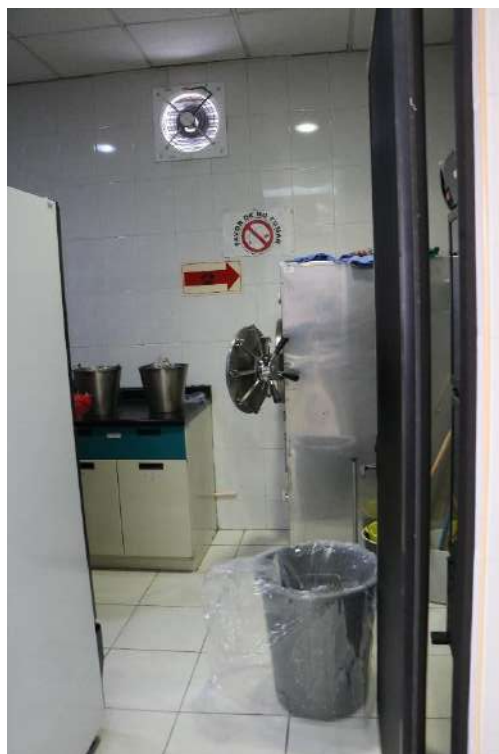
Figure 3. Identification of localized thermal and acoustic stress sources. The operation of high-pressure sterilization equipment contributes to ambient temperature elevation and increased background noise (dB) in adjacent work areas.
