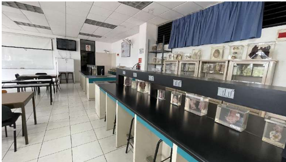
Figure 5. Anthropometric evaluation of fixed laboratory infrastructure. The height and depth of work surfaces present reach accessibility challenges for the 5th percentile of the female student population, inducing compensatory forced postures.
