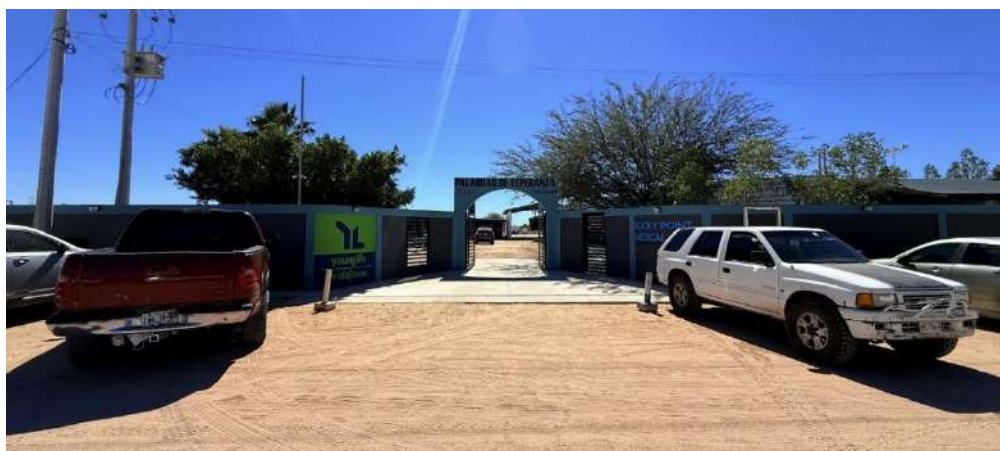
Figure 1. Front entrance to the community center.
