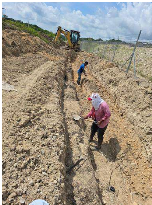
Figure 5 Workers digging trenches.
