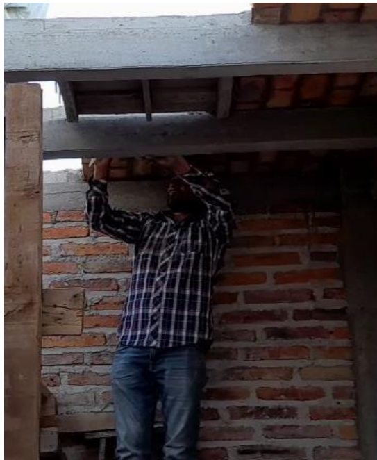
Figure 2. Vault ceiling cleaning
